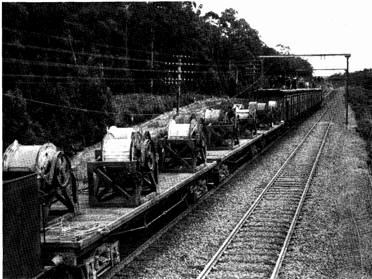
Erecting Overhead Wiring on a Duplicated Section of the Gippsland Line.
